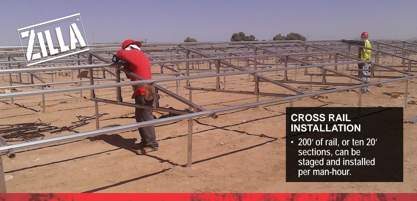
Cross rails simply attach to pre-fabricated trusses and are ready for module installation.
